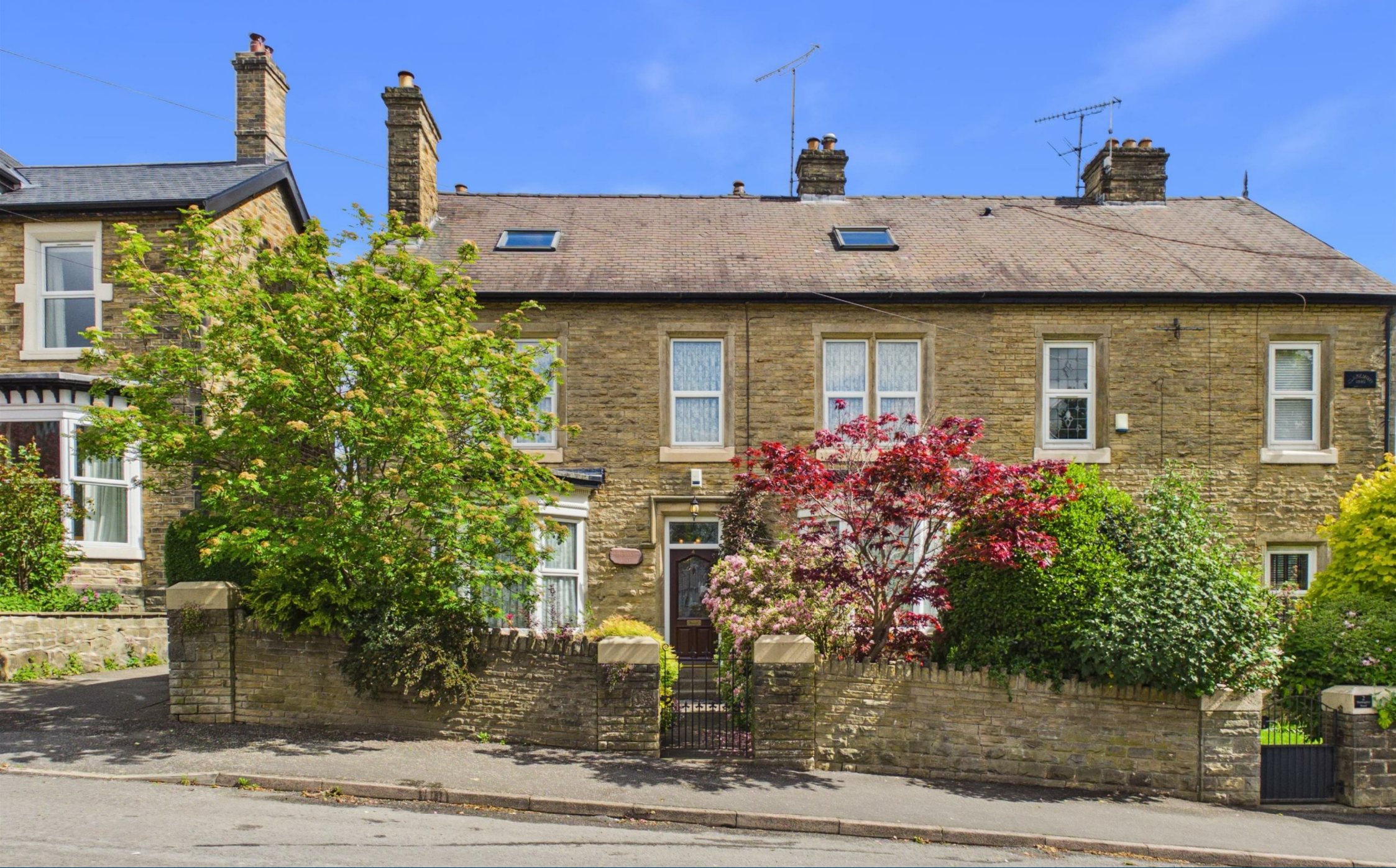
Mile Ash House, 4 Hartington Road, Millhouses, Sheffield, S7 2LE
